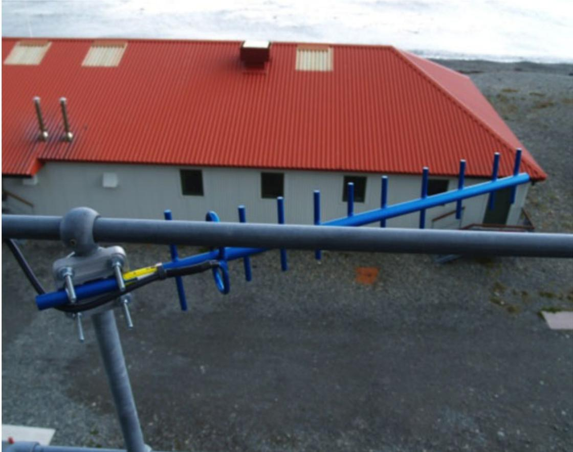
Figure 17: Yagi radio antenna on satellite tower opposite KEP communications room in the James Cook Laboratory.
