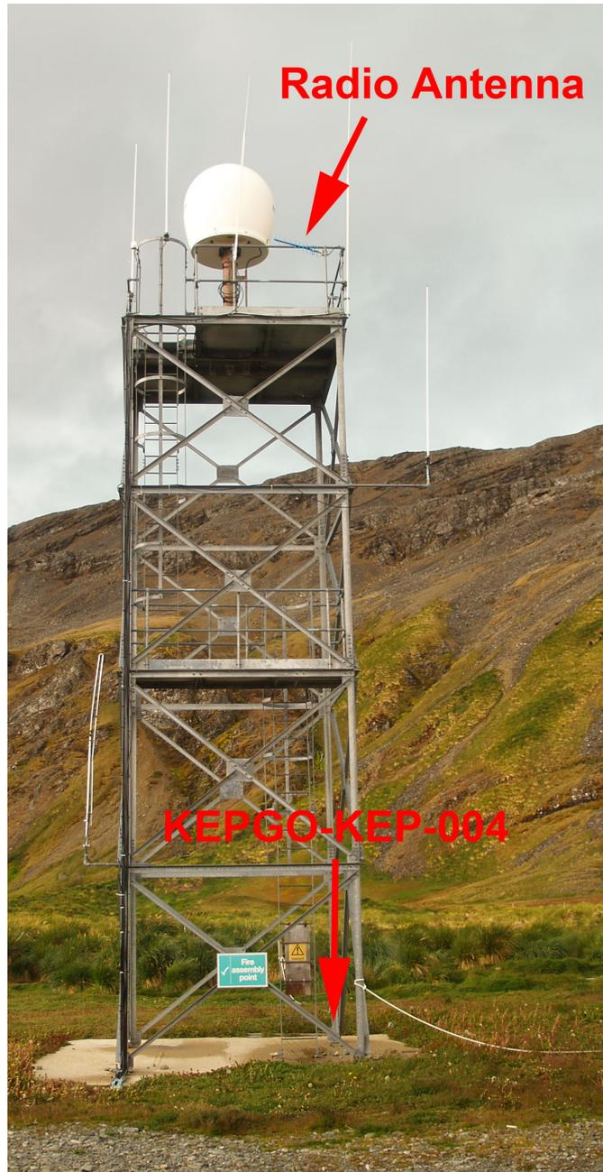
Figure 15: View of communication tower from communication room with receiving radio antenna and tide gauge benchmark KEPGO-KEP-004.
