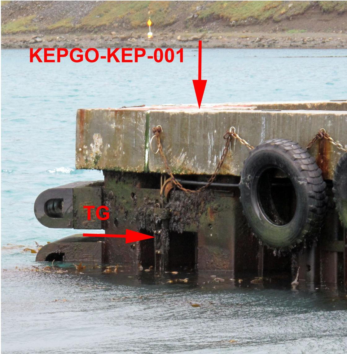
Figure 19: View of the jetty from slipway with tide gauge and TGBM KEPGO-KEP-001.
