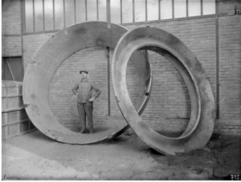
FIGURE 2.5 “Hauts Fourneaux. 1+1 anneau pour gueulard. Tintinger” (Blast furnace. 1+1 ring for blast furnace top. Tintinger). Undated. Digital positive from glass plate negative.
