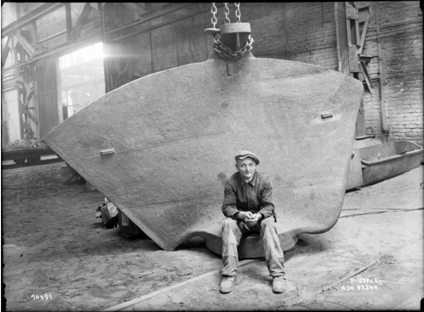
FIGURE 4.11 Worker sitting on a part of a hydraulic turbine. © INSTITUT EMILE METZ. CNA COLLECTION.
