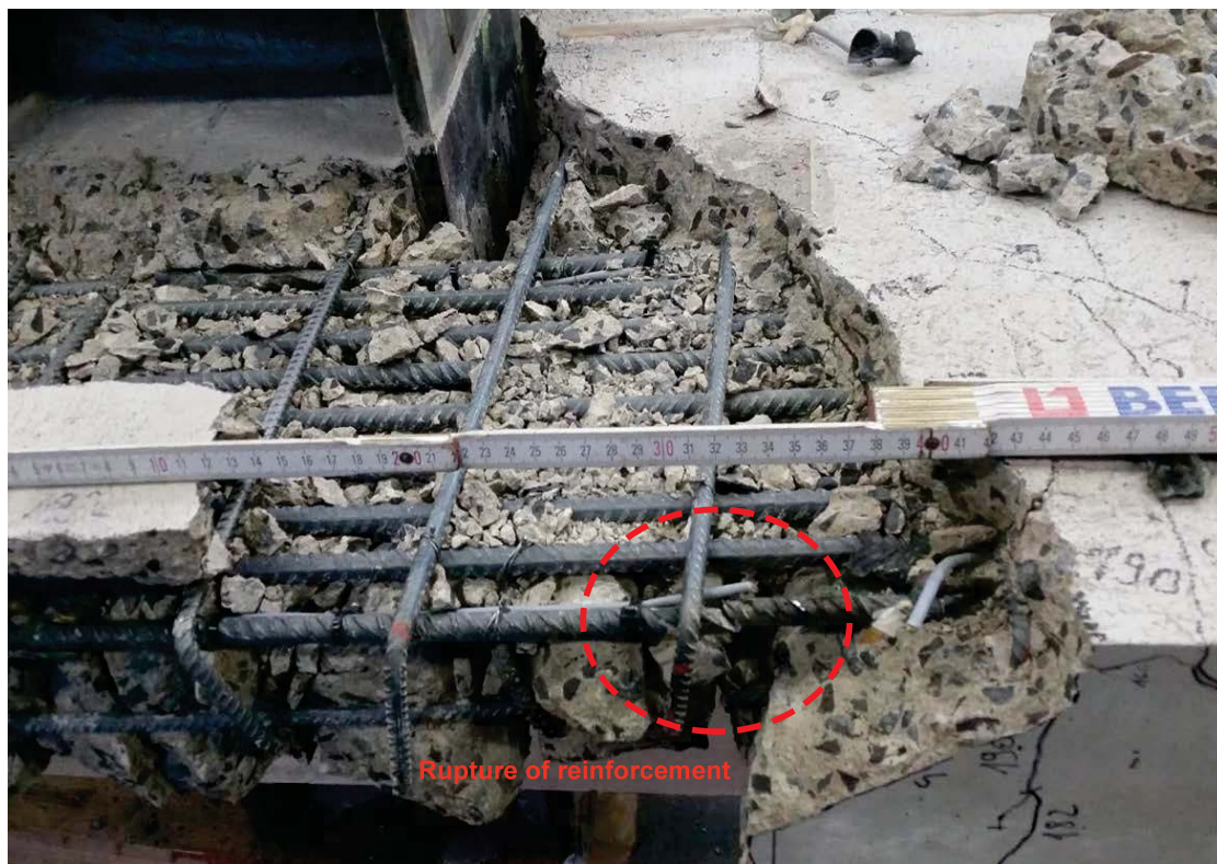
Figure 4.6: Rupture of reinforcement in test B21
