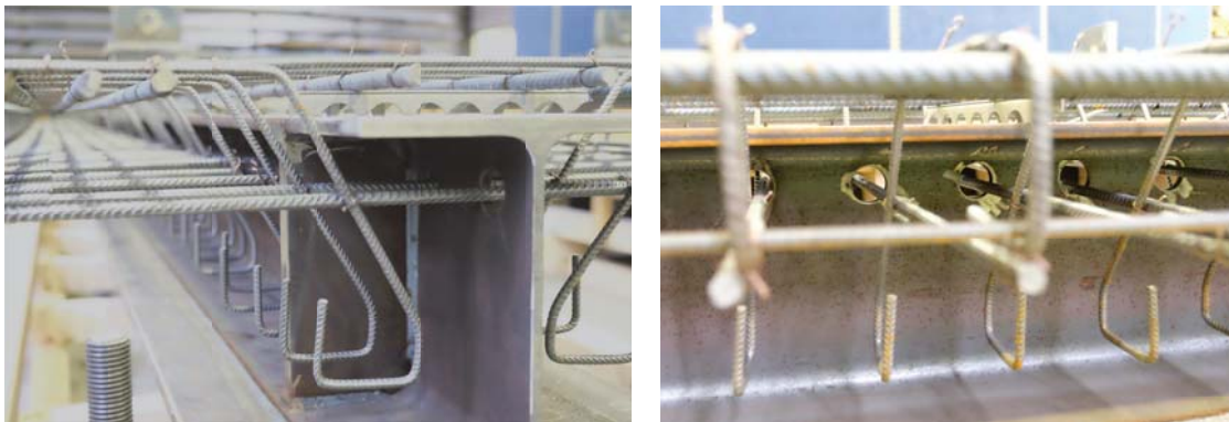
Figure 3.4: Dowel bars
