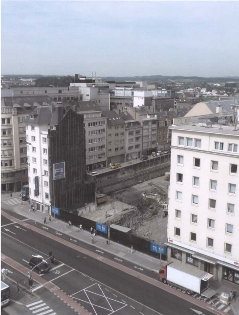
Figure 7.7. Demolition of the neighbouring building. Source: Mr Mertens' personal archive.
