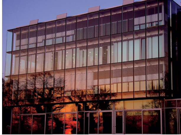
Figure 3.6: SSG façade of the Zeppelin University in Friedrichshafen, Germany, picture from Dow Corning Corporation (2010b)
