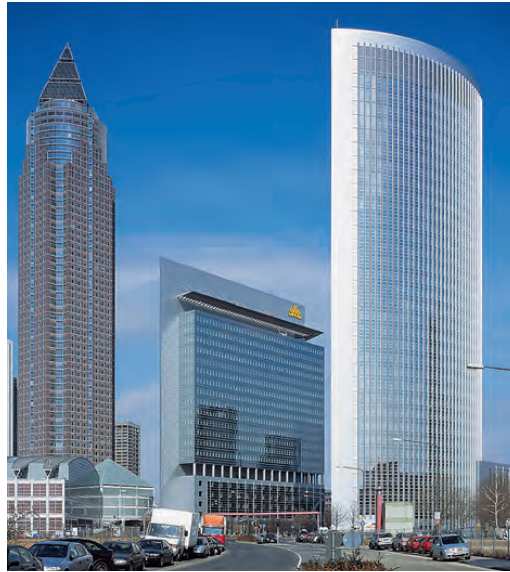
Figure 3.2: Example of a two-sided structural glazing system: Kastor (middle) and Pollux tower (right) in Frankfurt/Main (Germany), picture from Dow Corning Corporation (2010a)
