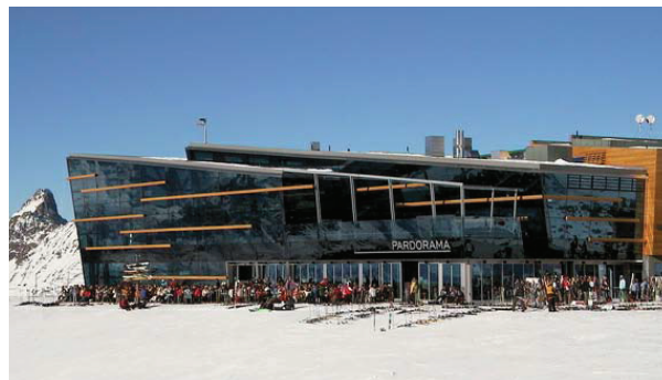
Figure 3.5: SSG façade of a restaurant in Austria, picture from Wolf (2010)
