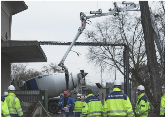
Figure 3.46: Truck mixer with concrete pump
