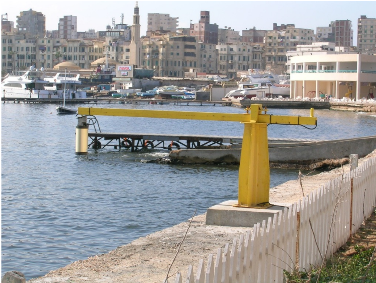
Radar tide gauge provided by NOC and UNESCO to Alexandria
