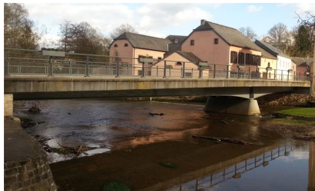
Figure 15. Bridge in Useldange in spring 2015
