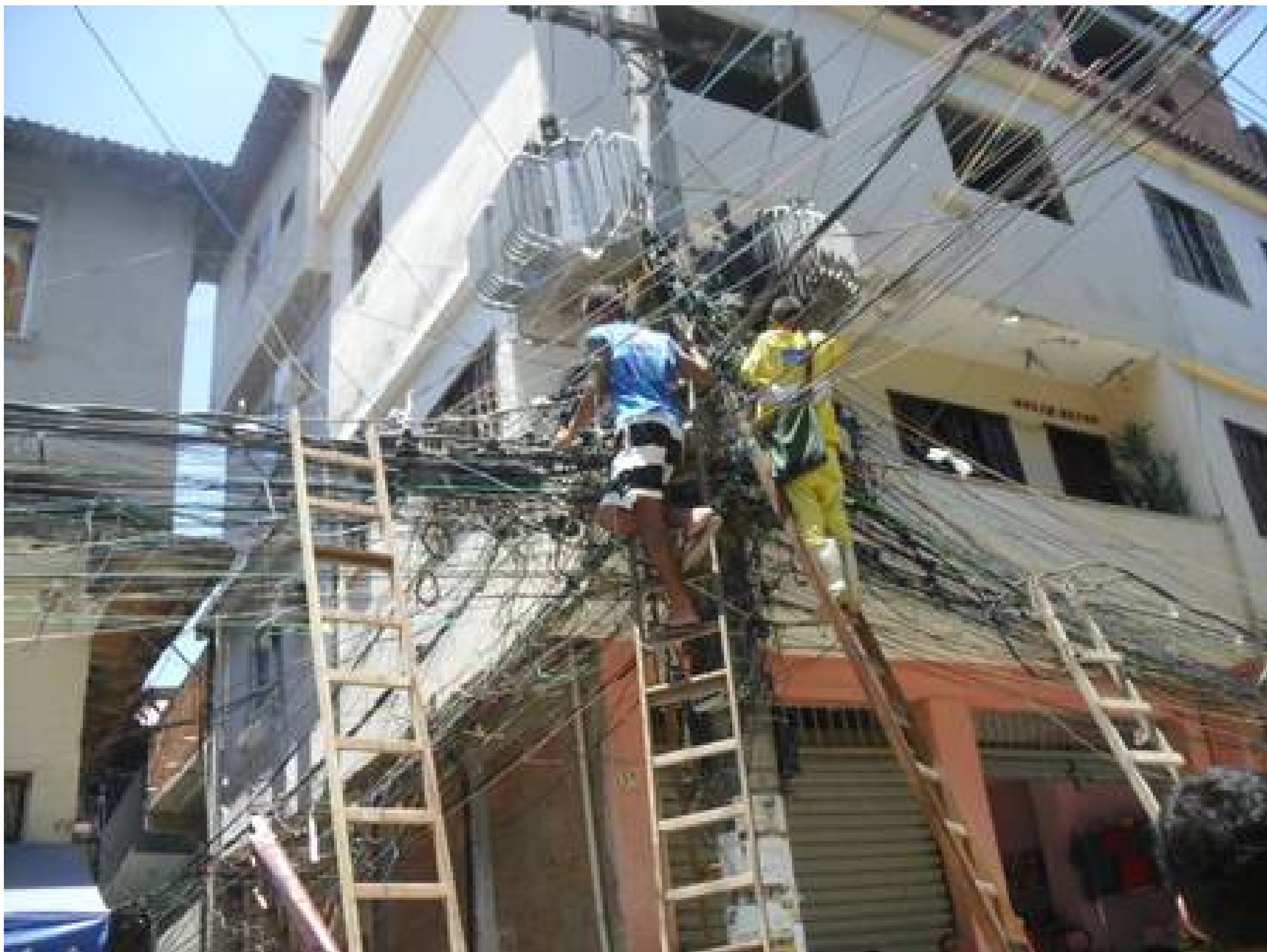
Fig. 1: That is what electricity theft looks 9 .
