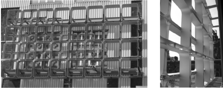
Figure 3: Mock-up of the fixed external façade element in front of an existing test room
